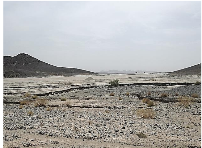
Fig. 1. A view of the tailing dame of Qaleh-Zari copper mine
